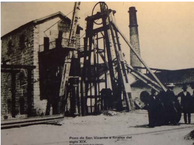
Fig. 3 Photograph of the original state from the engine house of Cornish pumping installed in the San Vicente well at the end of nineteenth century in the Interpretation Centre of Mining Landscape Linares (Jaen).
