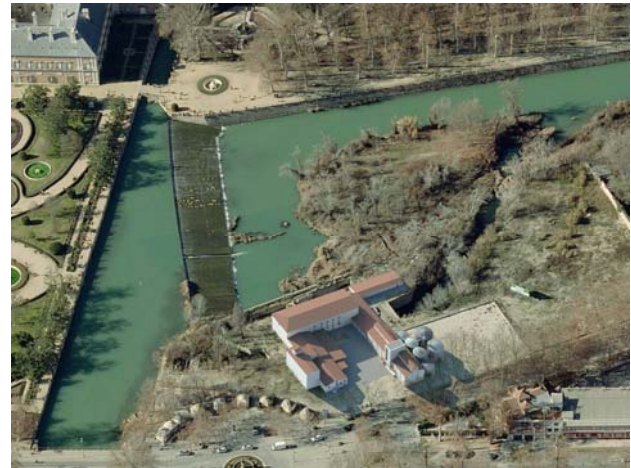
Fig. 17 West view rebuilt on BING montage.
