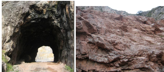
Fig. 3 Old railway tunnel and jointed rock mass in the area
