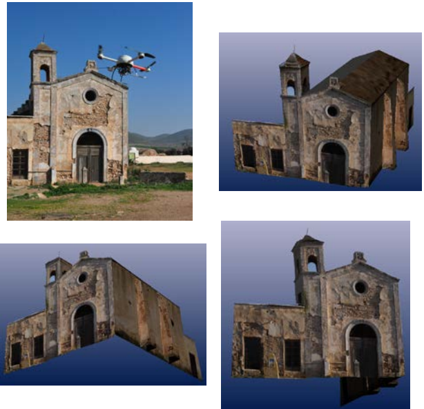
Fig. 11 a) Actual image of the Chapel in “Cortijo del Fraile”. b), c) and d) Points of view of the photogrammetric model of the Chapel.
